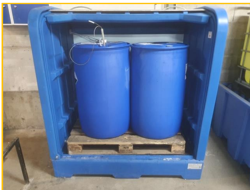
Figure 2 : Stockage acide sulfurique
